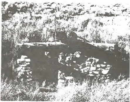
Figure 88. Stone and log structure which comprises site 5RB438. This site is located on tract 1, west of Piceance Creek.
